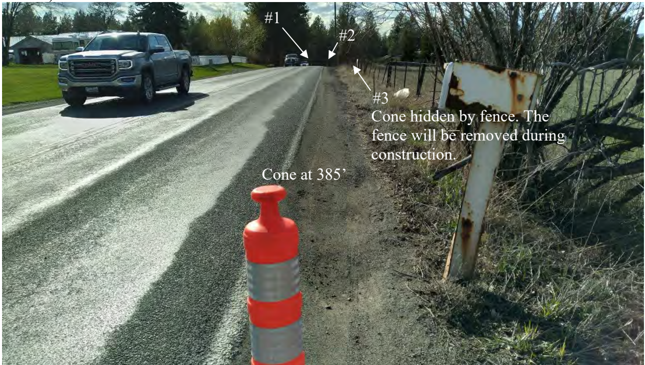
Photo 3 – Looking west from Cone at 385' to the intersection of Galaway Road (South Access) & 32 nd Avenue
